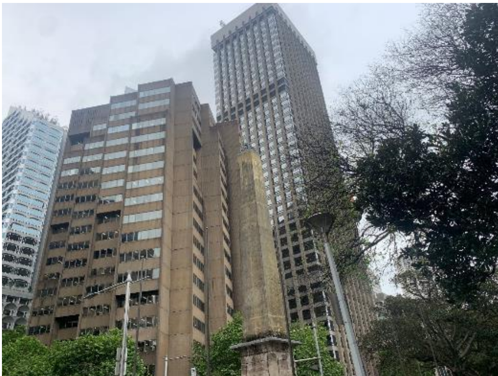
Figure 8: Elizabeth Street frontage, view from Hyde Park. Adjoining building to south is the former Producers and Citizens Life, later Aetna Life building 1974, by Roy Grounds and Co and Cheeseman Doley Brabham and Neighbour joint architects..
