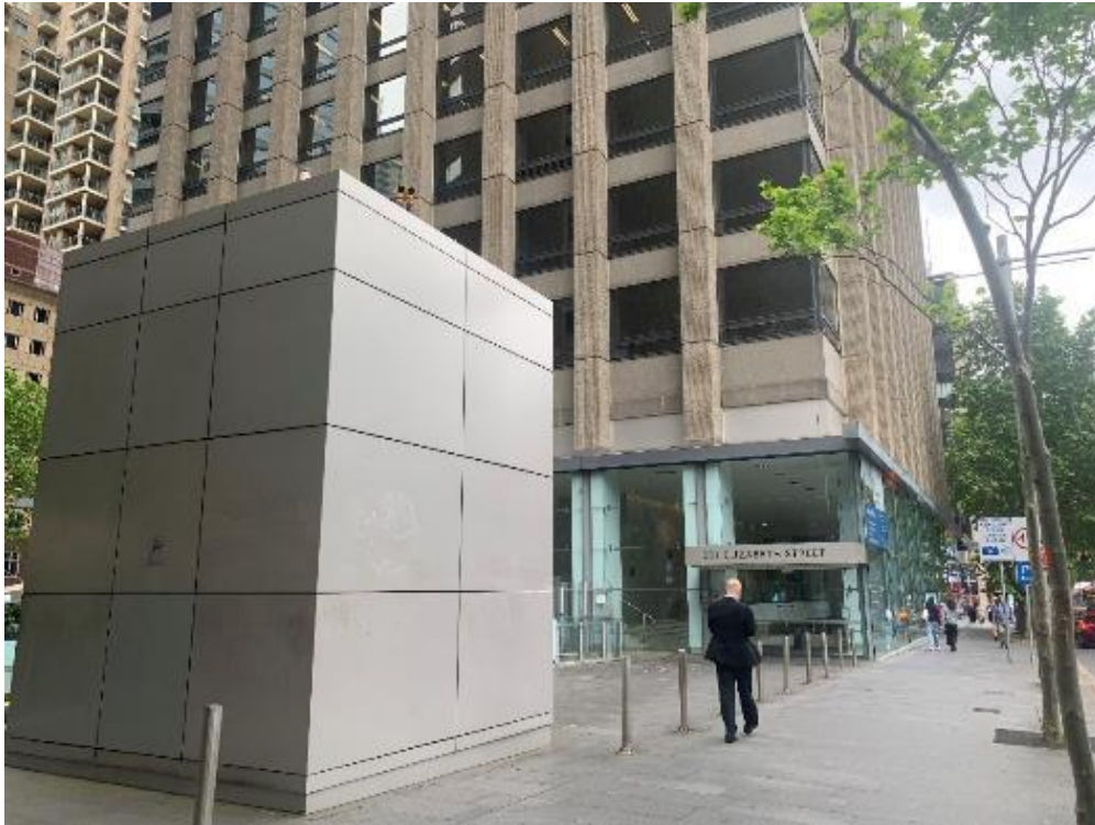
Figure 7: Site's Elizabeth Street frontage, view facing north-west
