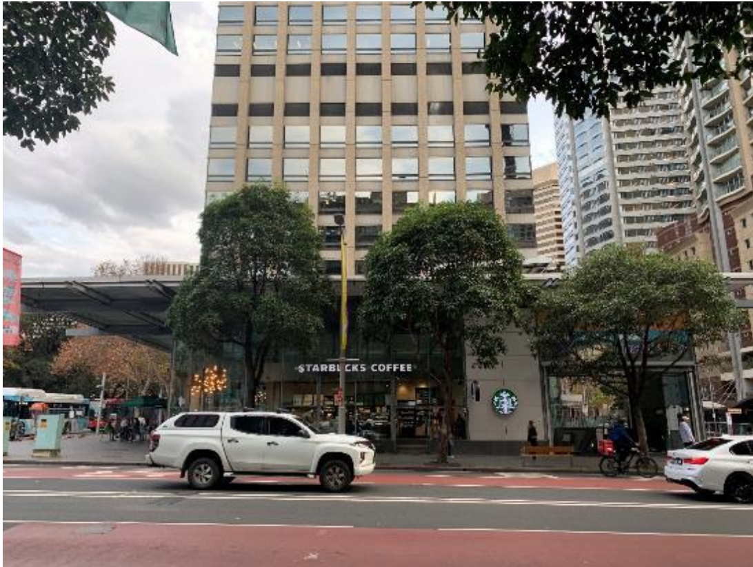
Figure 5: Site's Park Street frontage, view facing south
