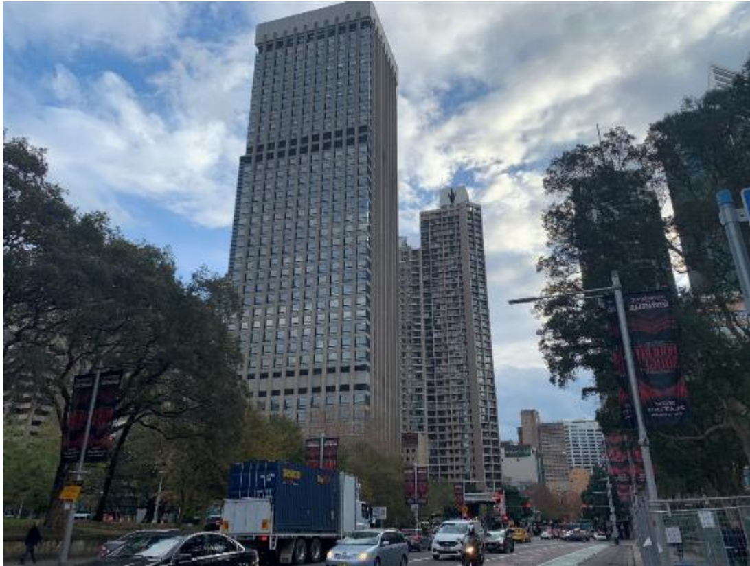
Figure 3: Existing tower, view from Park Street facing west
