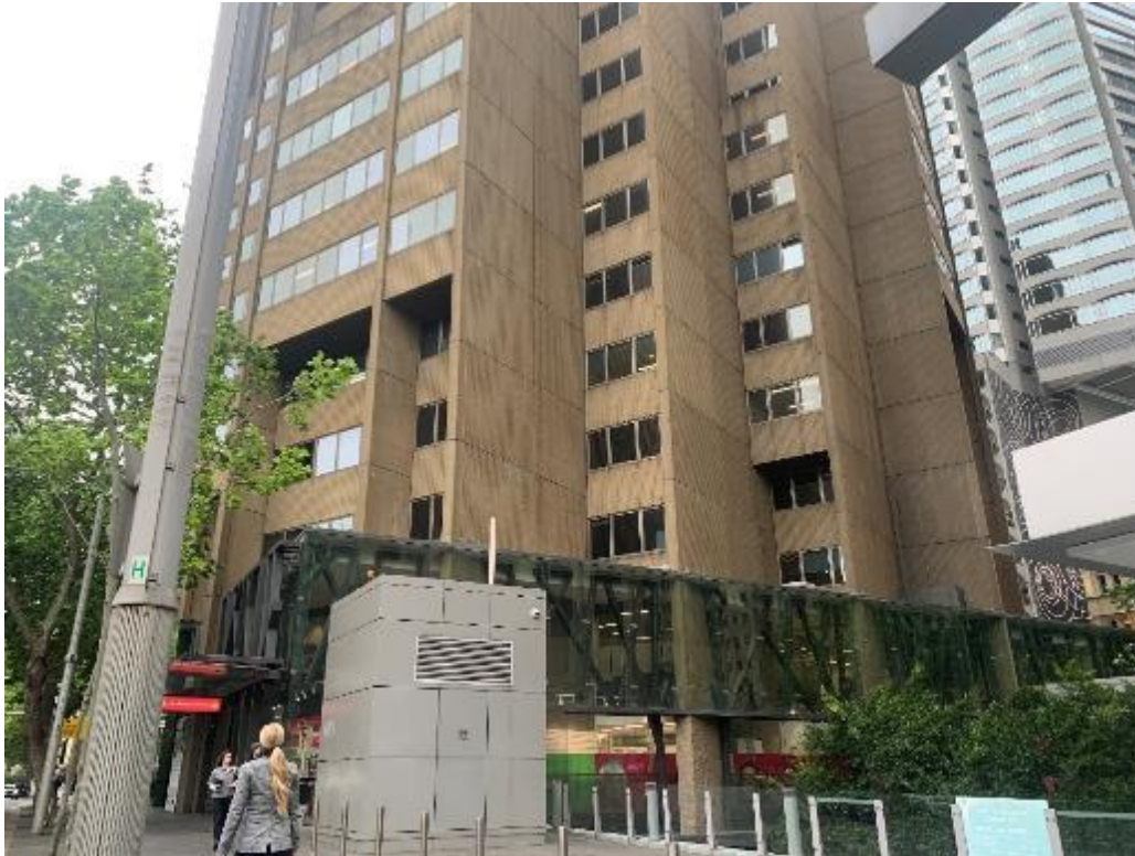
Figure 9: Site's southern frontage. Adjoining building to south (219-227 Elizabeth St) shown.
